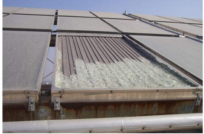
Fig. 7: Broken Glasses and Dust Accumulation
